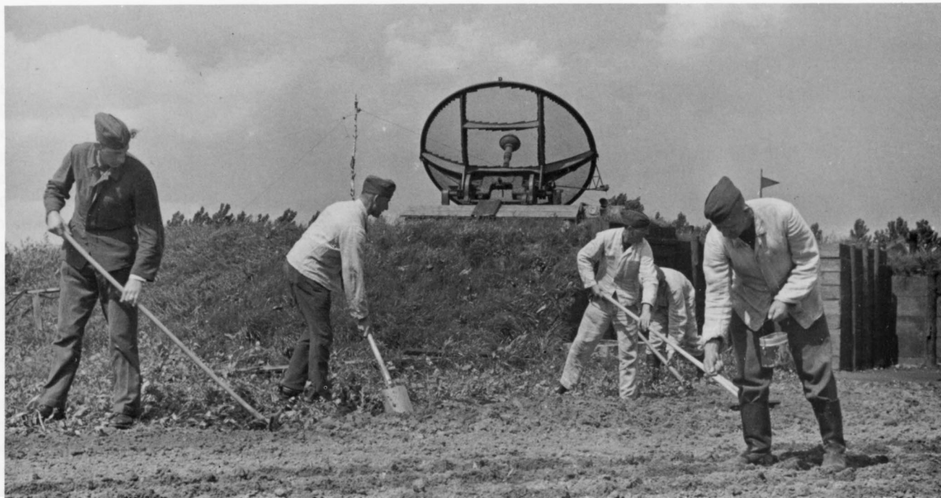
Above: This Mannheim crew is carefully working on enriching their cooking pot by planting vegetables around their radar site. On the right side of and linked to the FuMG 64's reflector is an sighting collimator. The radar controller could use this sight to direct the crew to a target which he'd acquired optically. He also had his own scope available to him for monitoring the crew, which showed ranging and direction finding data.
