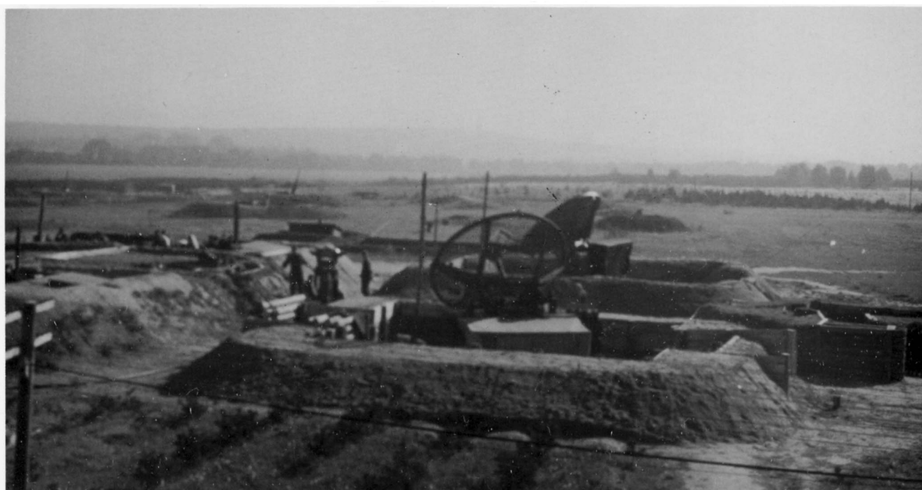
Below: The two FuMG 64 Mannheim and 62 Würzburg systems here are sited in the well constructed facilities of a 88 mm heavy battery, of which a few guns can be seen in the background. The earthworks around the FuMG had a diameter of around 8 meters and a height of 1.8 to 1.9 meters. This prevented interference from height finding errors and the system was able to function without the so-called "bottom lip" (see next page). A Flakrichtgerät 40 A anti-aircraft control system with its two collimators can be seen next to the radar sites.
