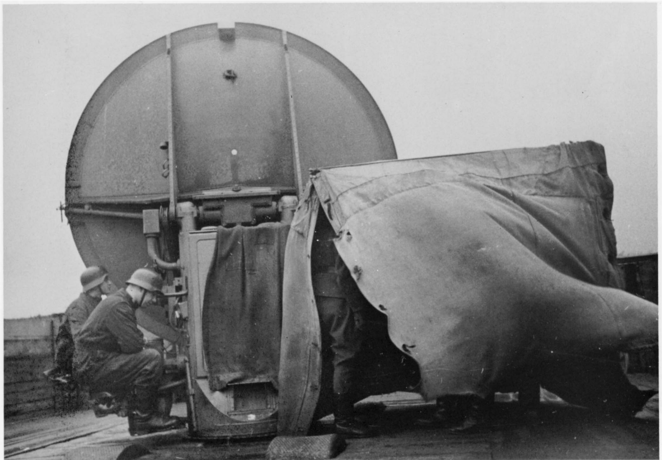
Protected by a canvas cover, the B1 is at work on the CRT of the precision ranging system, the B2 is at the horizontal tracking scope and the B3 at the vertical tracking scope.
