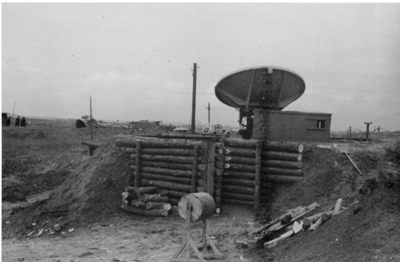
Below: This is probably the site of a prototype system. The dish is the same style as the small Würzburg A-, B-, C- and D-systems. Based on scale comparisons with the wooden support wall (which has a height of approx. 1.90 m - 2.30 m) and the vehicle, it appears that the diameter of the antenna dish would be larger than 3 meters, possibly the 4.5 meter type as on the FuMG 68 Ansbach. The light colored speck on the upper edge of the dish is an anchor point for a larger IFF antenna. In the background to the left is a 150 cm searchlight.
