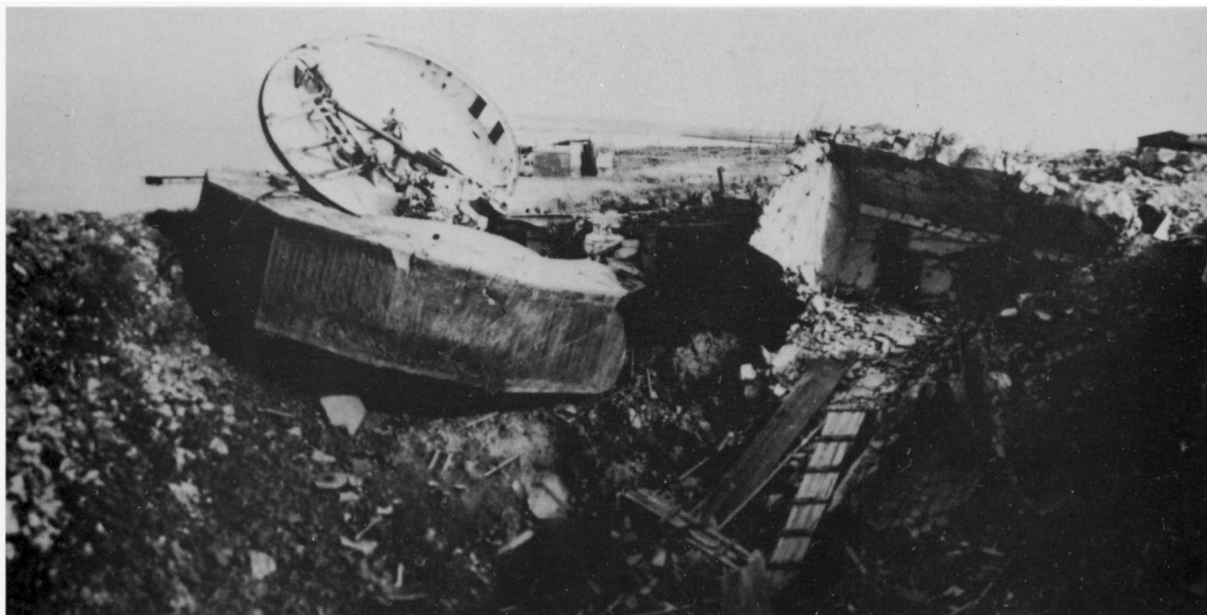
Above: A bombed out radar of 3/M.F.I.A. 242 on the island of Heligoland following the raid of 18 April 1945. This probably was a Würzburg-Riese, which along with its entire bunker took a direct hit.
