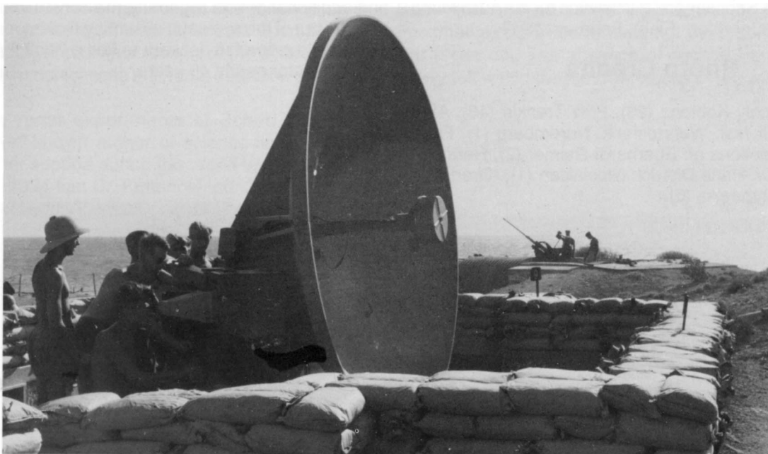
FuMG 39 T along the Atlantic seawall in southern France. A 20 mm Flak 38 can be seen in place in the background, its purpose to protect the site against strafing attacks.
